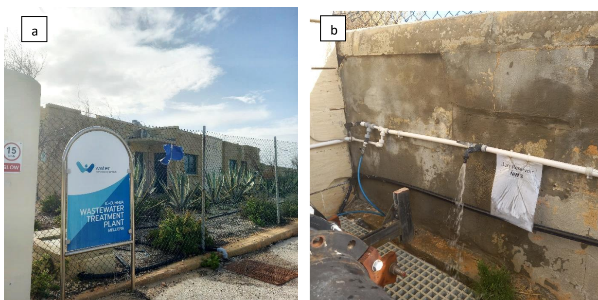
Figure 19 (a,b) Ċumnija Wastewater Treatment Plant
